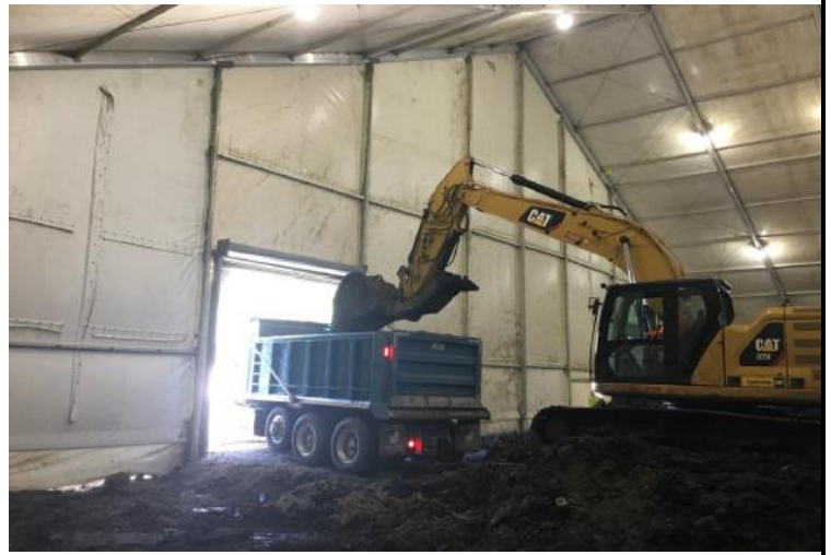
Loading Material into Trucks
