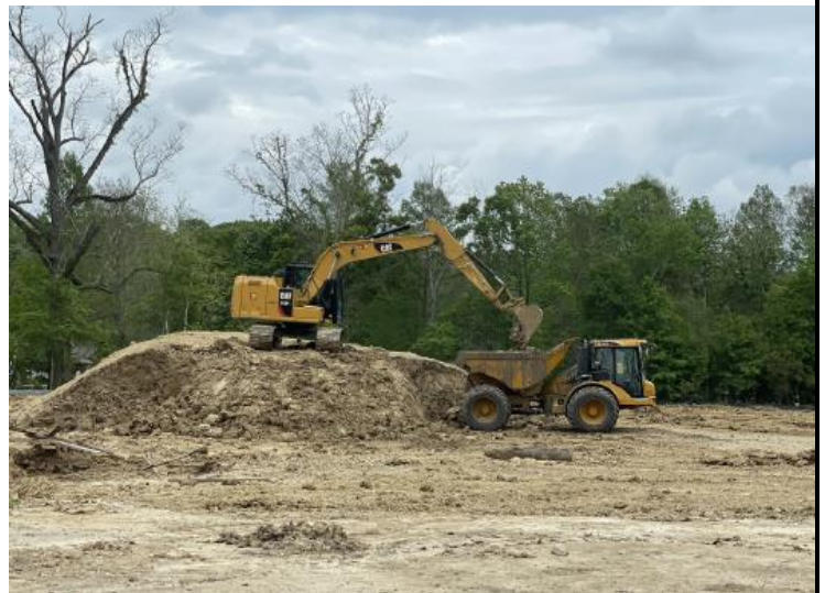
Transporting Clean Backfill to Excavation
