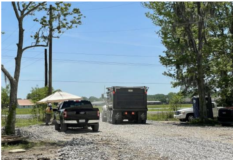
Loaded Trucks Leaving the Site for the Landfill
